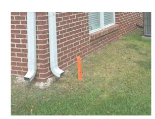
UH-1 / UH-2 INSTALLATION LOCATION WILL BE MARKED BY A STAKE AND/OR PAINT, CSPIRE/ OSP WILL INSTALL CONDUIT 8" UNDERGROUND TO DESIRABLE UH-1 LOCATION.
